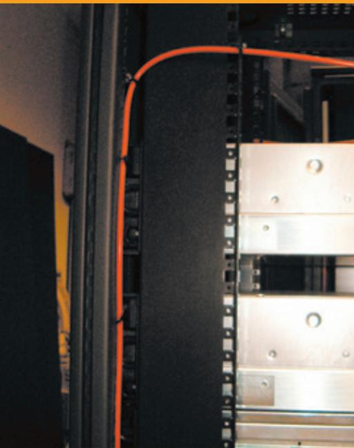
The flexible red Firetrace Detection Tubing will quickly and reliably detect and suppress a fire at its source.
